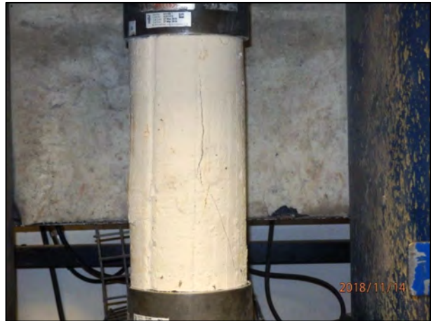
Rear view (post-test)
